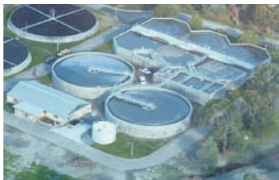
Figure 8.7 An aerial view of a sewage plant
